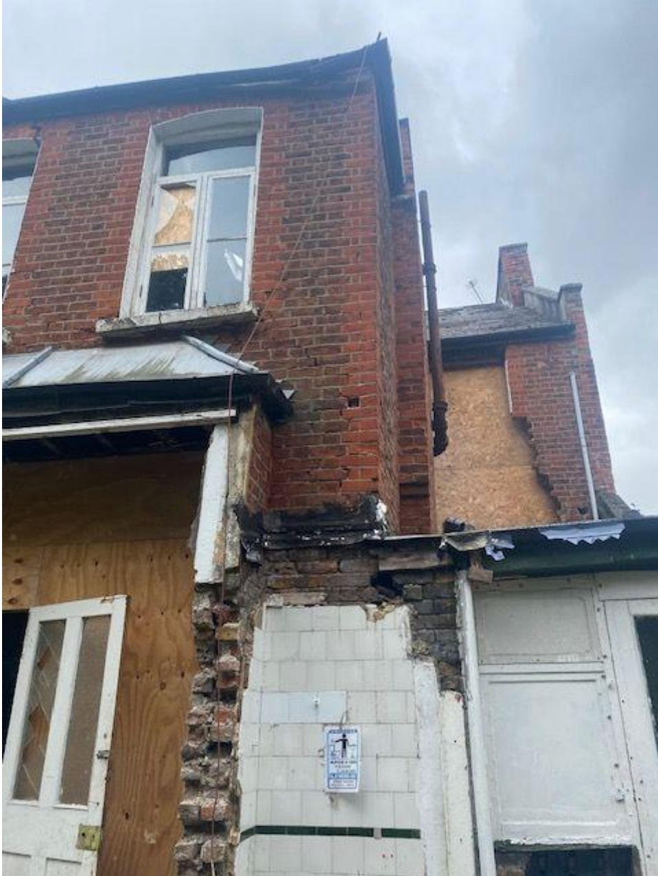
View of site (rear)
